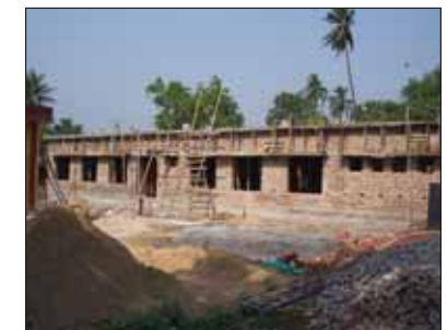
a BPHC being upgraded
